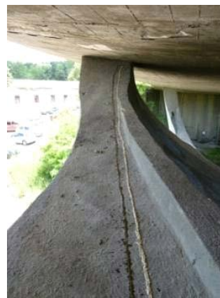
Optic fiber sensor for strain monitoring
